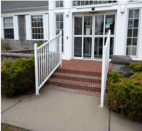
Stairway , Handrails : Handrail Extension not Parallel
