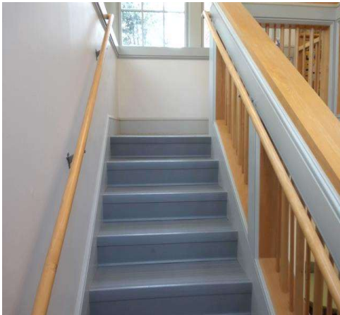
Stairway , Handrails : No Top Handrail Extension
