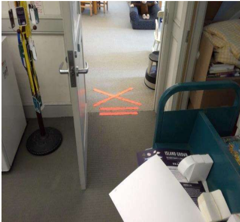
Door , Latch Side Clearance : Front Approach Latch Side Clearance
